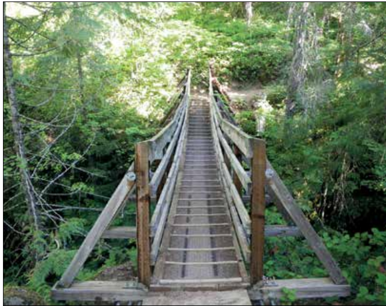
The hike to Falls Creek Falls includes several footbridges.
